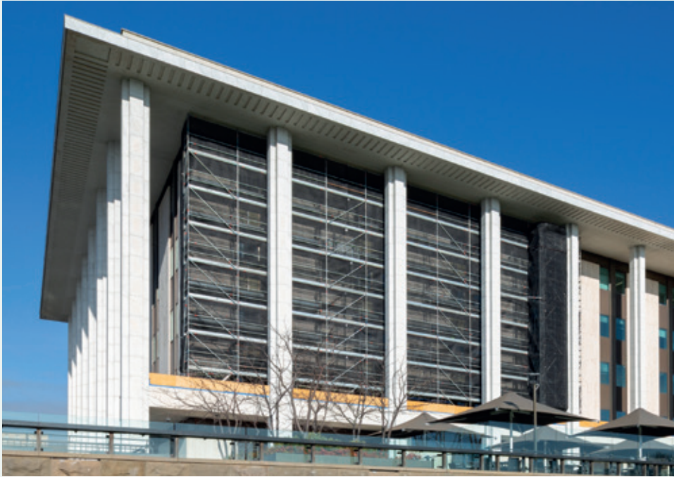
The Library's heritage windows covered in scaffolding.
